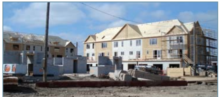
Construction is progressing at Daniels FirstHome™ Eglinton West
