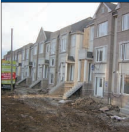
Phase Two Under Construction
